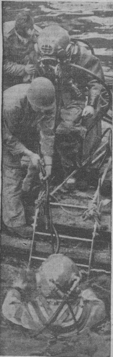
Two under-water GIs, members of an engineer and port construction repair group, wear air-conditioned steel helmets as they go down into a French harbor. Their mission is to police barnacles from concrete forms. Just released by the censor, this picture was taken early in the campaign on the continent.
