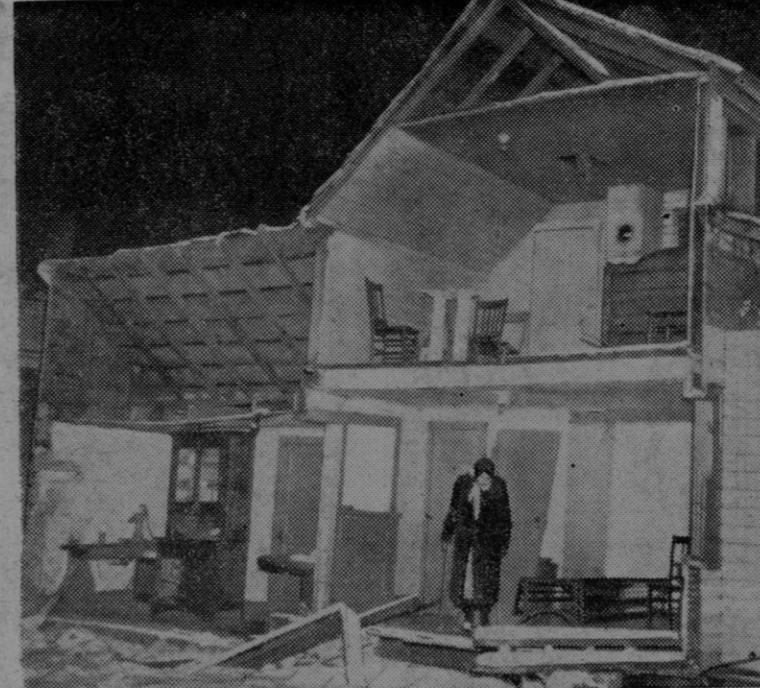
When Mrs. Clara Casprzyk, a crippled widow, refused offers to have her dwelling moved to make way for a street-widening project in Silver Lake, Minn., the town council ordered the house sawed in half. Mrs. Casprzyk, shown emerging from the bisected building, continues to live in one room of the house which was untouched by the carpenters' saws.
