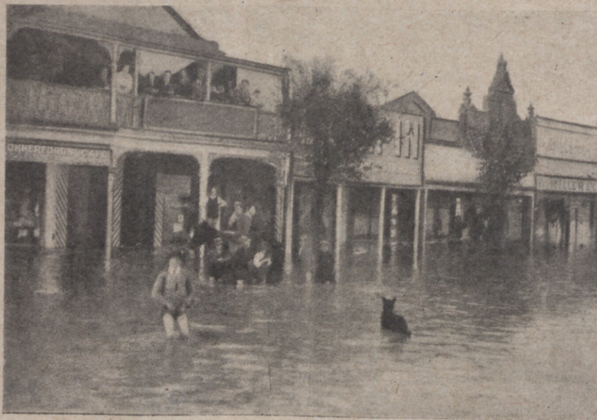
Bridge Street, Benalla (Vic.) during the May floods.
