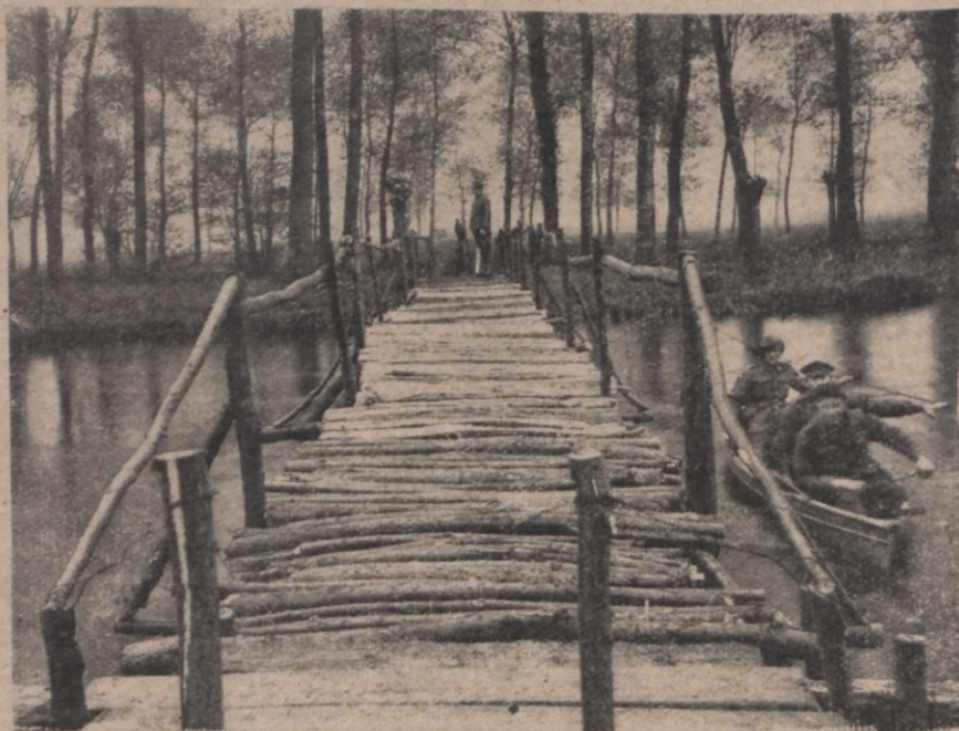
A temporary bridge built of materials found near at hand.
