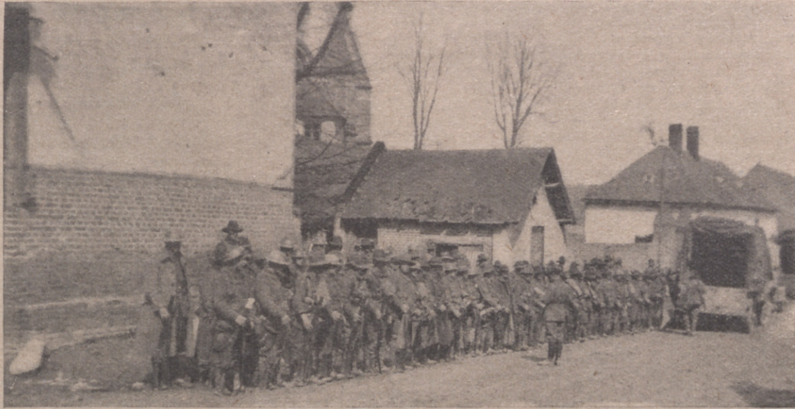
Australian Tunnelling Corps setting out to wire a new Defence Line.
