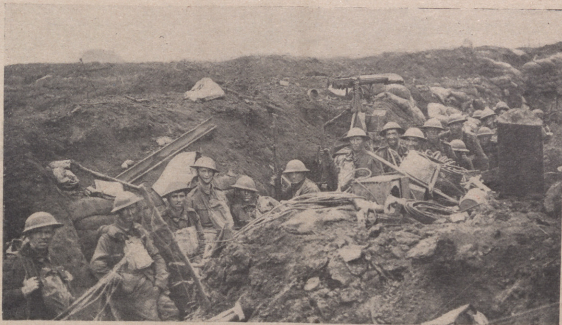
A First Line Trench.
