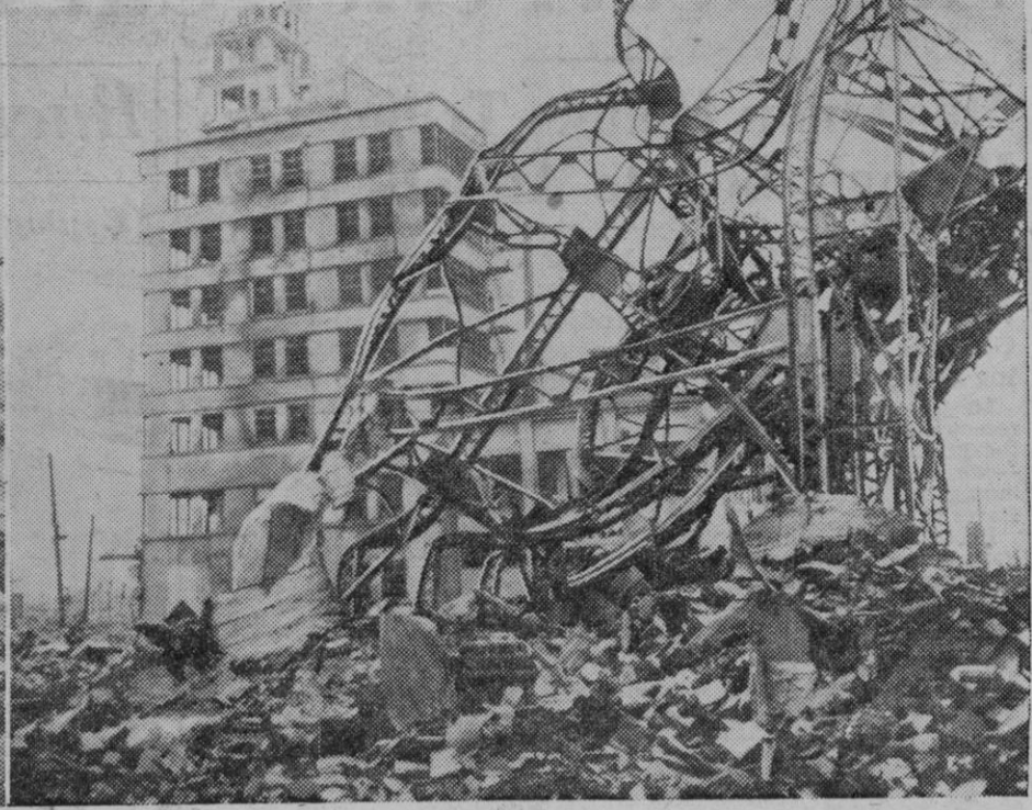
Twisted in a pattern of destruction is this mass of tangled girders—the steel framework of what once was a modern building in downtown Hiroshima. The structure in the background, although still standing, is windowless and gutted by flames.
