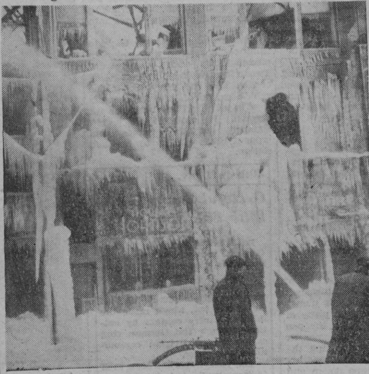
A 36-hour play of water upon a smouldering fire which gutted two three-story buildings on So. Salina Street, Syracuse, left this icy display. Damage was estimated at $100,000.
