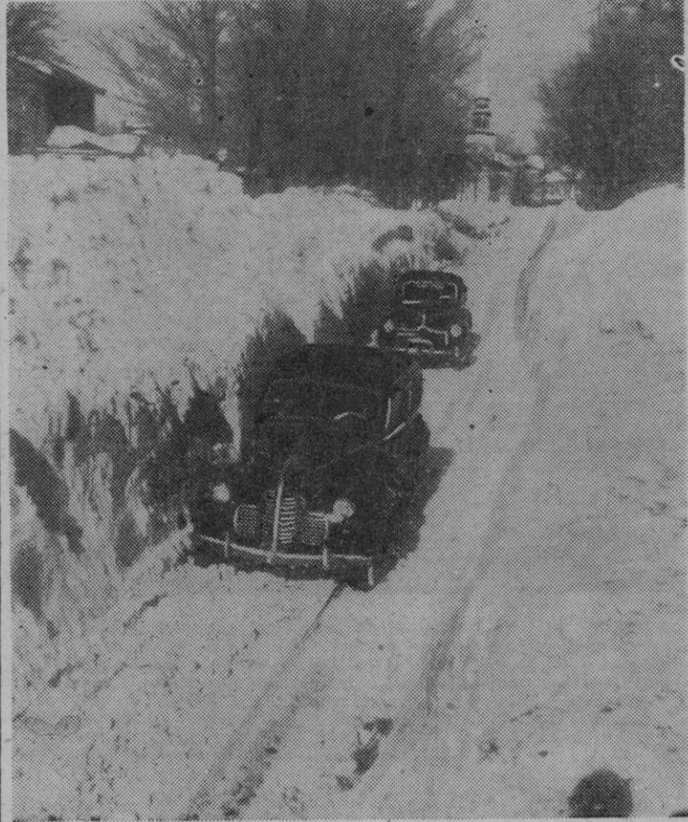
Pompey, a village in Onondaga County, N.Y., almost found itself in the position of ancient Pompeii—except that the up-state village had to contend with snow instead of lava. Here's U.S. Highway 20, looking east into little Pompey, which has almost finished its job of cutting through big snowdrifts.
