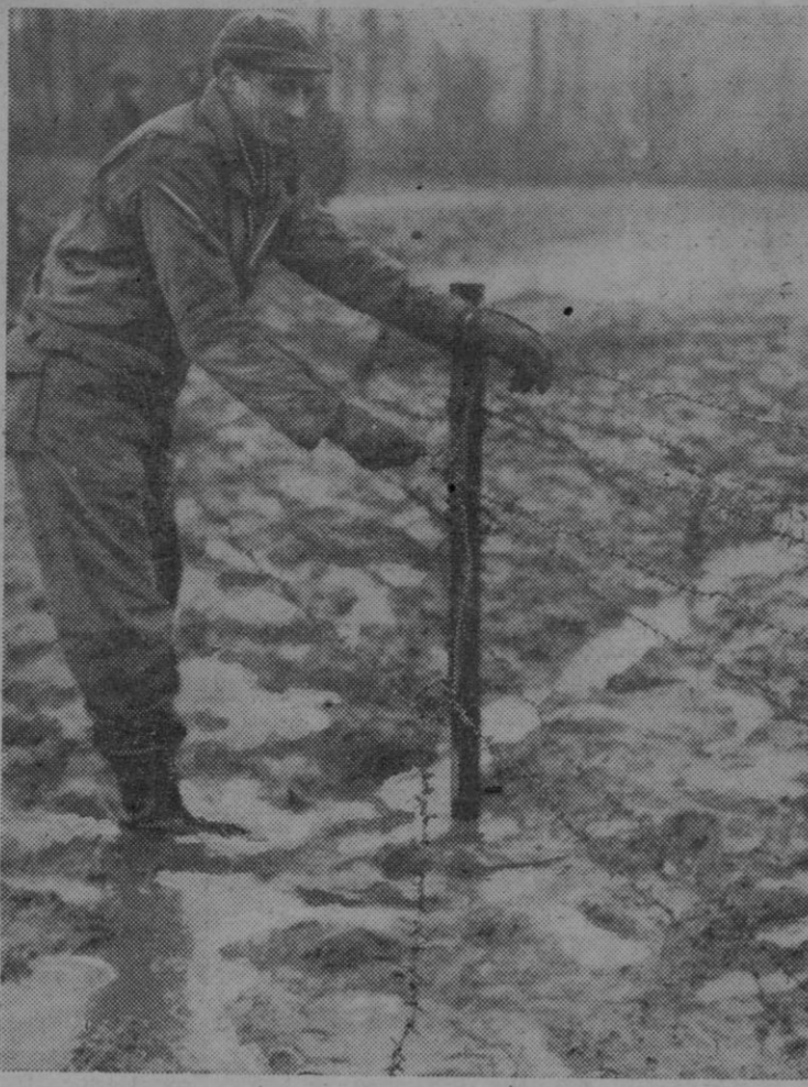
U.S. Army engineer completes fastening of "apron" for a barbed-wire entanglement in Hatmat, France. Mud made work difficult but assured a sturdy setup when ground hardens.
