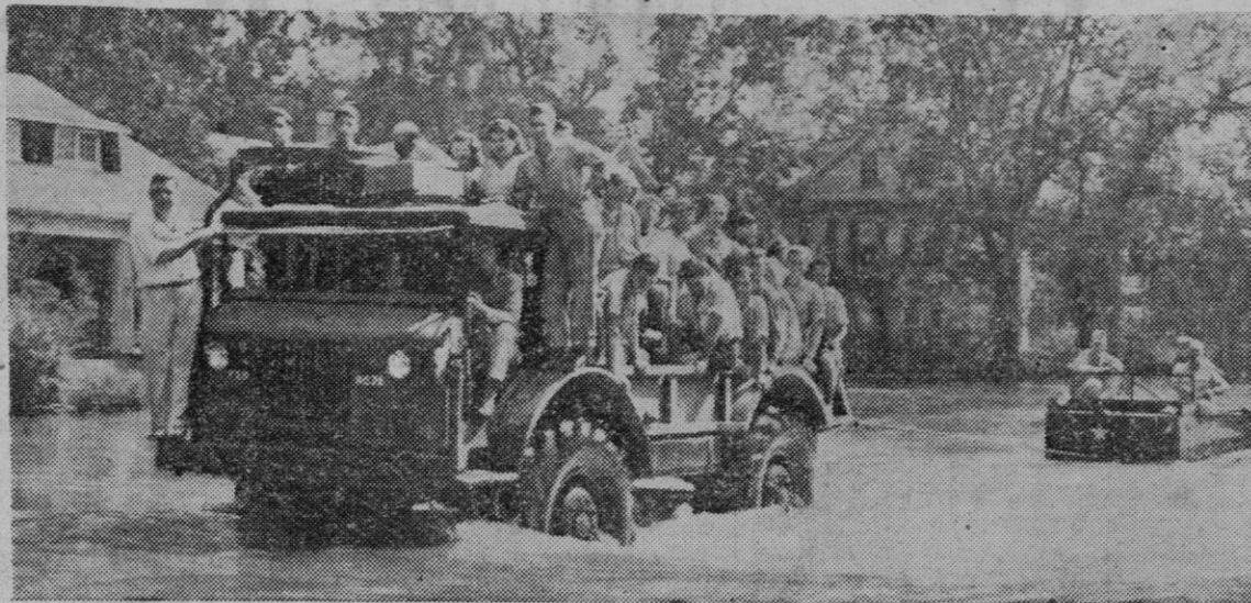
Hub-deep in floodwaters of the rain-swollen Cape Fear River, an Army truck hauls a load of refugees from an inundated area of Fayetteville, N.Y., to higher ground, where an evacuation hospital has been set up to take care of the homeless. The GI truck is towing a weasel that stalled.
