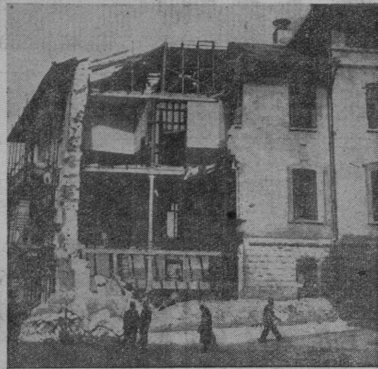
For the second time in 22 months, terrorists placed a bomb in the police headquarters at Jerusalem, with the results shown above. Six were killed and two escaped.
