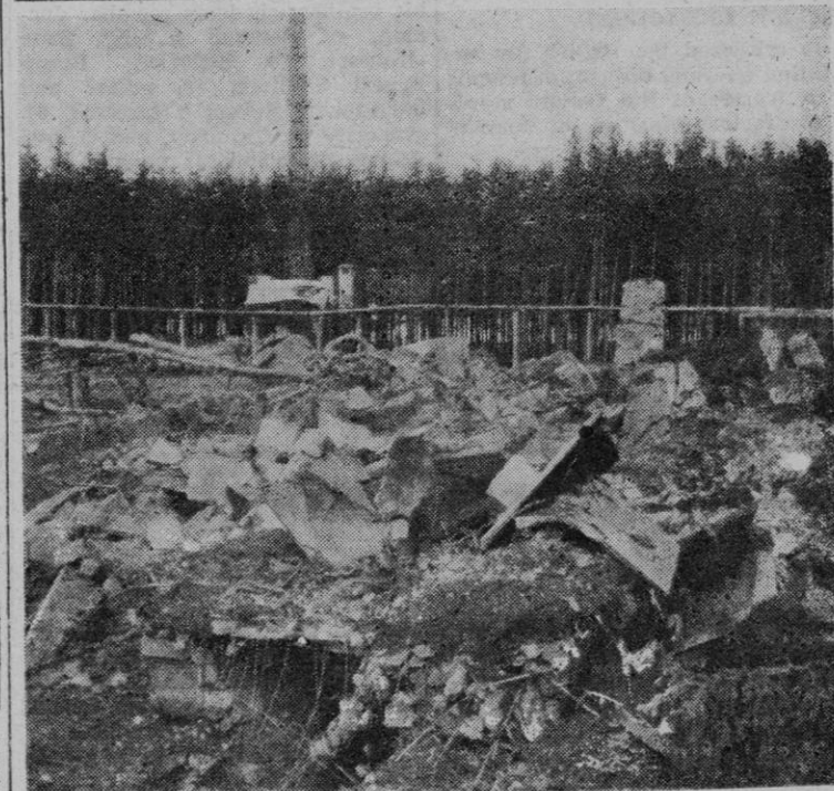
LAST BLAST: A smokestack and a heap of rubble are all that indicate where the recently destroyed giant German munitions factory at Kaufbeuren once stood. It was blown up by the XX Corps Engineers, U. S. Third Army, as part of the U. S. demolition program for Germany's war potential.
