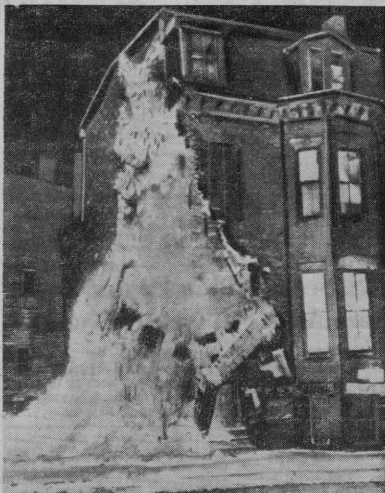
With a roar, the side of an apartment building caved-in in Boston. Occupants of the building had been warned in advance and there were no casualties.
