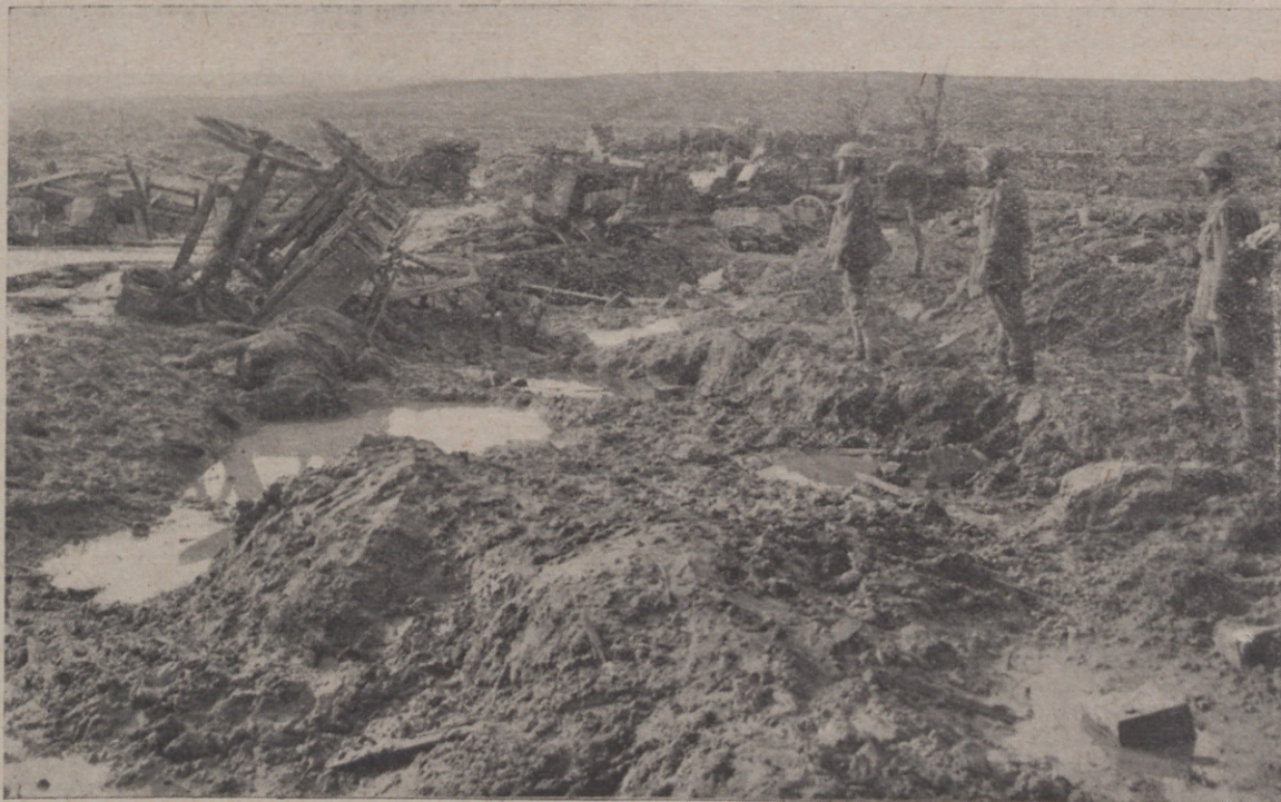
A corduroy track littered with the ruins of war transport.
