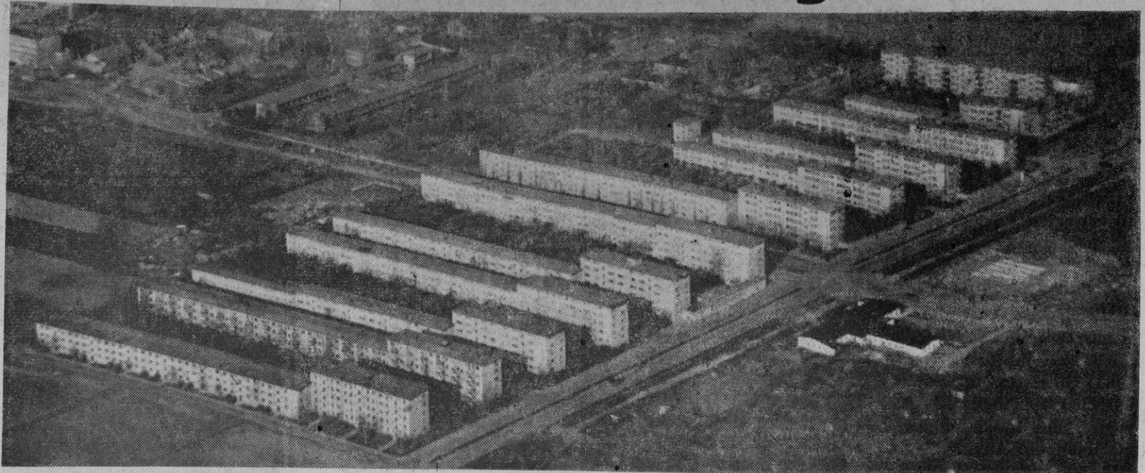
AIR VIEW showing the housing project established in Frankfurt to provide homes for families of U. S. Army personnel.
