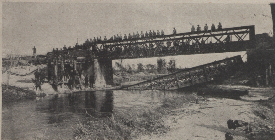
This bridge—completely wrecked—was repaired by Australian Pioneers in six days.
