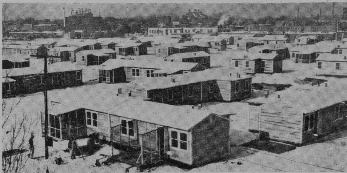
HOMES FOR VETS: Acting to help solve the housing shortage, the Massachusetts Institute of Technology is constructing 100 houses near Memorial Drive in Boston for married veterans who are returning to the institution to study. It is a 430,000-dollar project. The houses will be ready in March.
