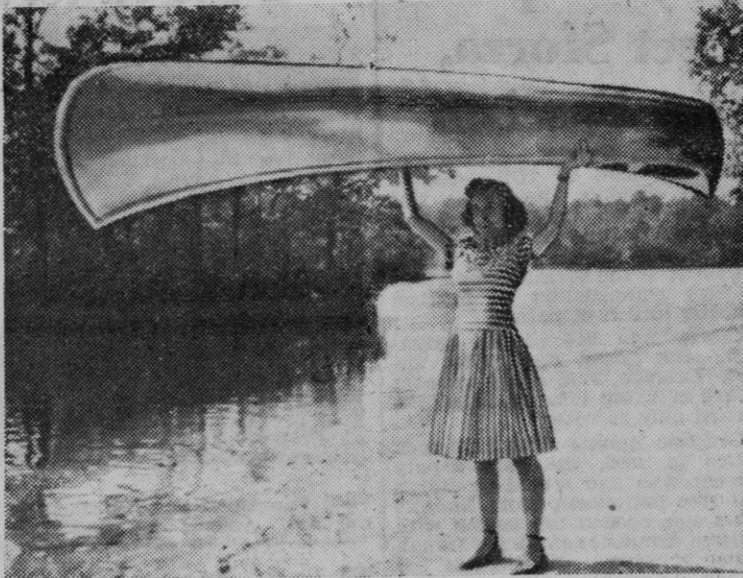
Looks like a circus strongwoman act, but the canoe Joy Lesavage is hoisting weighs only 38 pounds. The all-aluminum craft is being made as a sideline by the Grumman Aircraft plant in Bethpage, L.I.
