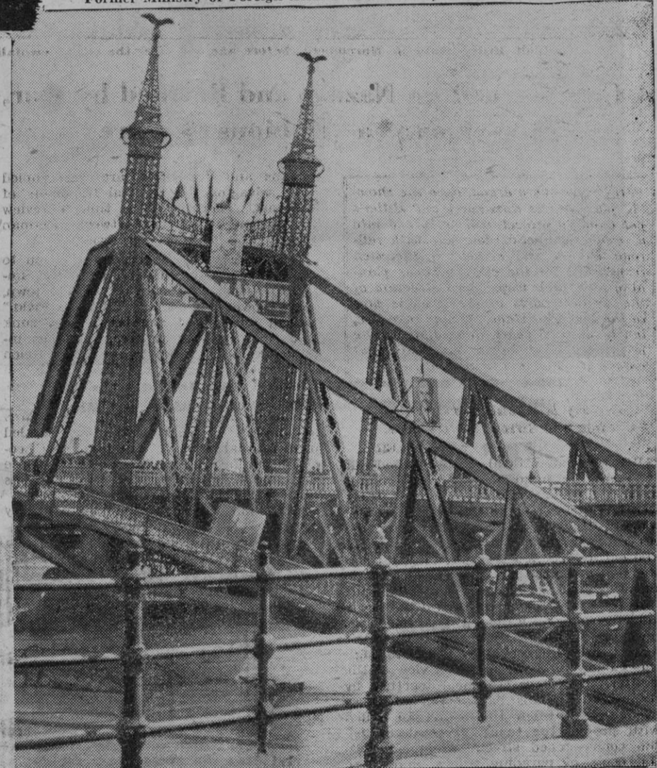
Franz Josef Bridge, linking Buda with Pest, has been repaired by Russian engineers. Hungarians await freezing of Danube with fear, know that bridge's pilings will block ice and bring floods to city.
