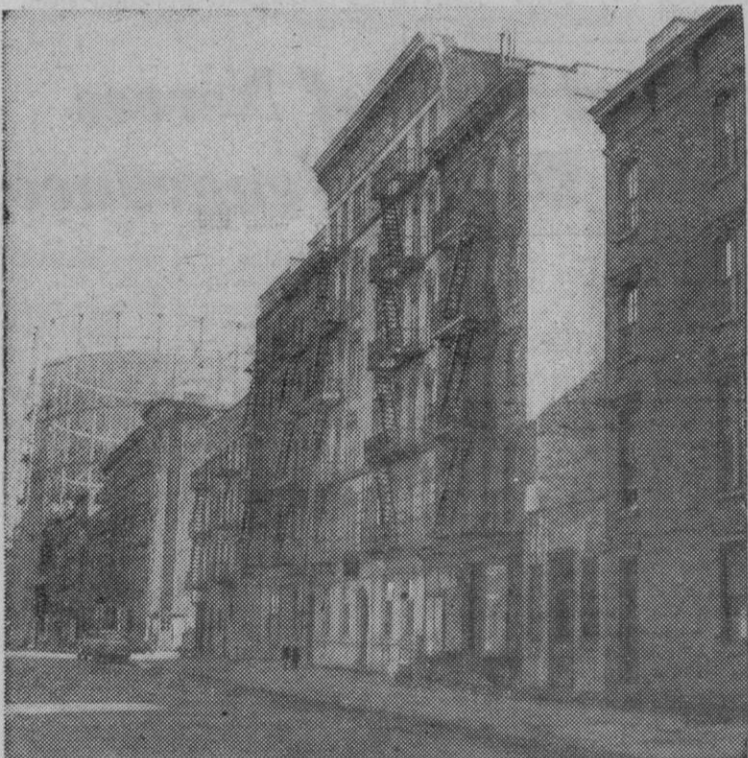
The famous—or rather, odoriferous—gashouse district in old New York will be torn down to make way for Stuyvesant Town, a private postwar housing project. Here is a street scene at 16th street and Avenue B, looking east... and one of the gas tanks down the street.
