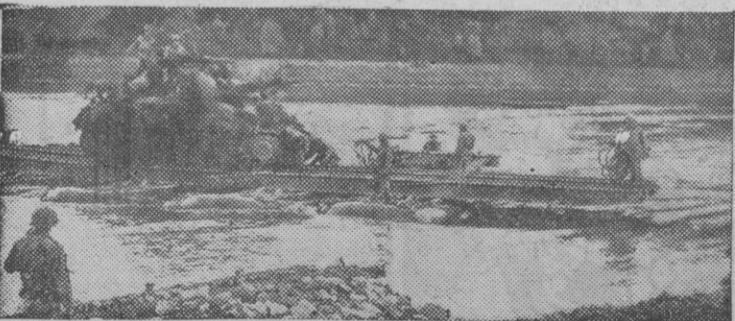
The army's M-1 treadway raft, loaded with an American medium tank, spans a stream in Belgium. The raft, which looks like a floating bridge, is propelled by flat-bottomed motorboats.
