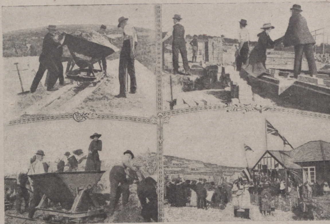
Sunday voluntary workers at Matraville, near Maroubra Beach, Sydney, where 150 cottages are being built for returned soldiers.
