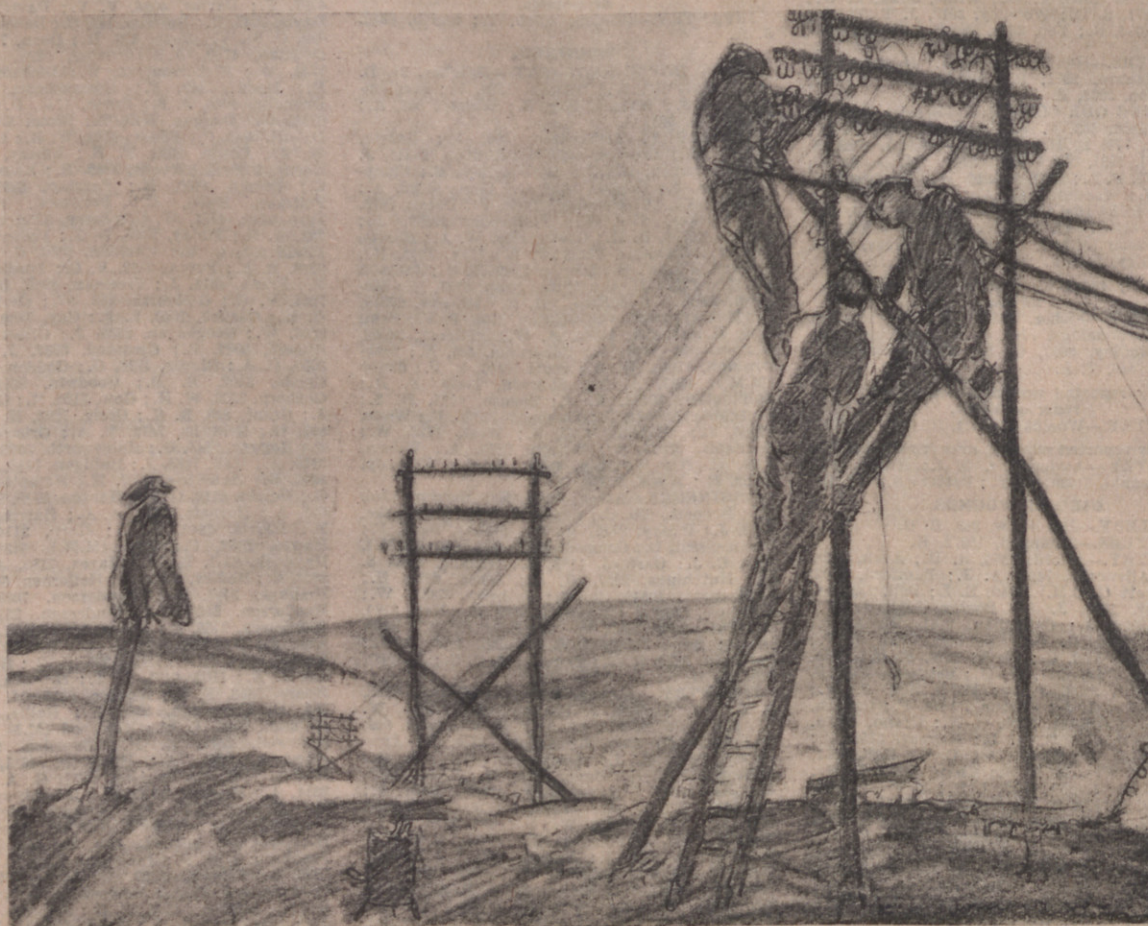
Mending the wires at Wolff Huts, Pozières.
