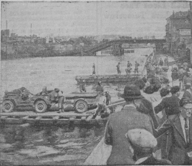
American jeep crosses the Oise River near Compiègne, France, on raft propelled by ropes from opposite shore. In background is main bridge, wrecked by Germans before they fled town.
