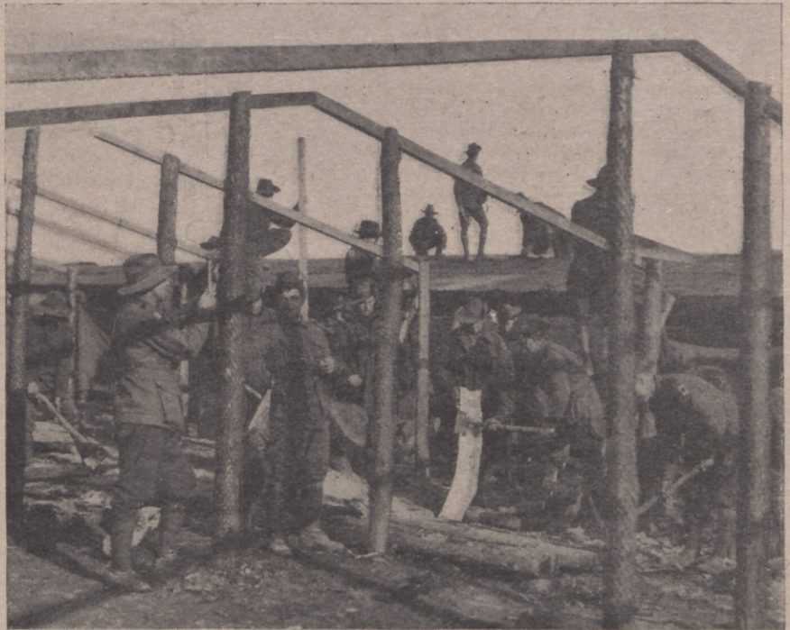
Australian Pioneers build shelters for the horses during winter. It is necessary to wire-net the posts so as to prevent the horses from chewing them.
