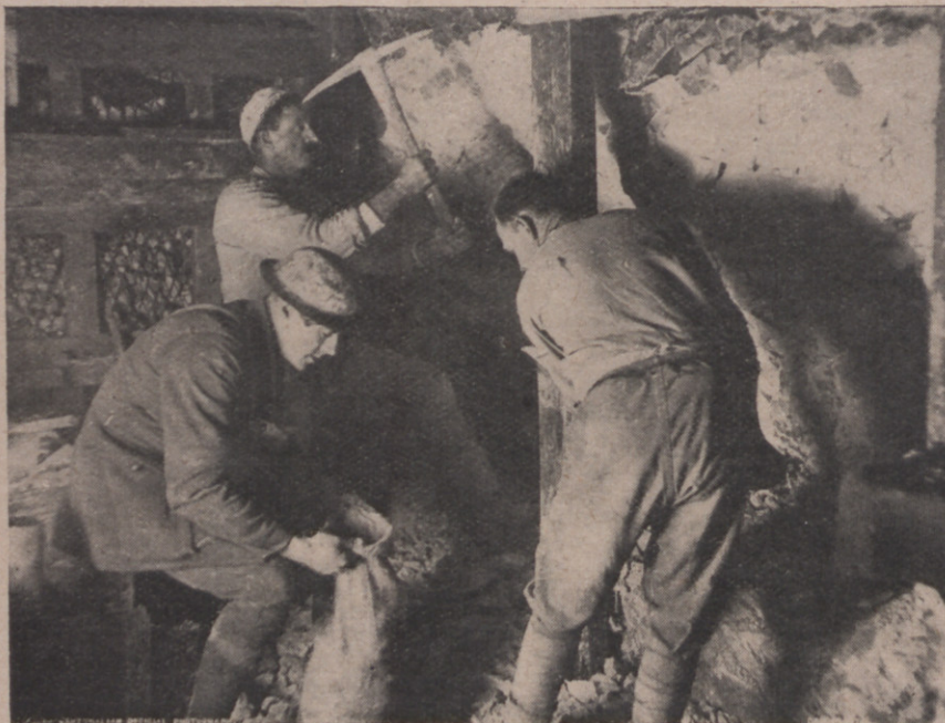
An Australian Tunnelling Company constructing an underground dug-out. (Australian Official Photograph.)
