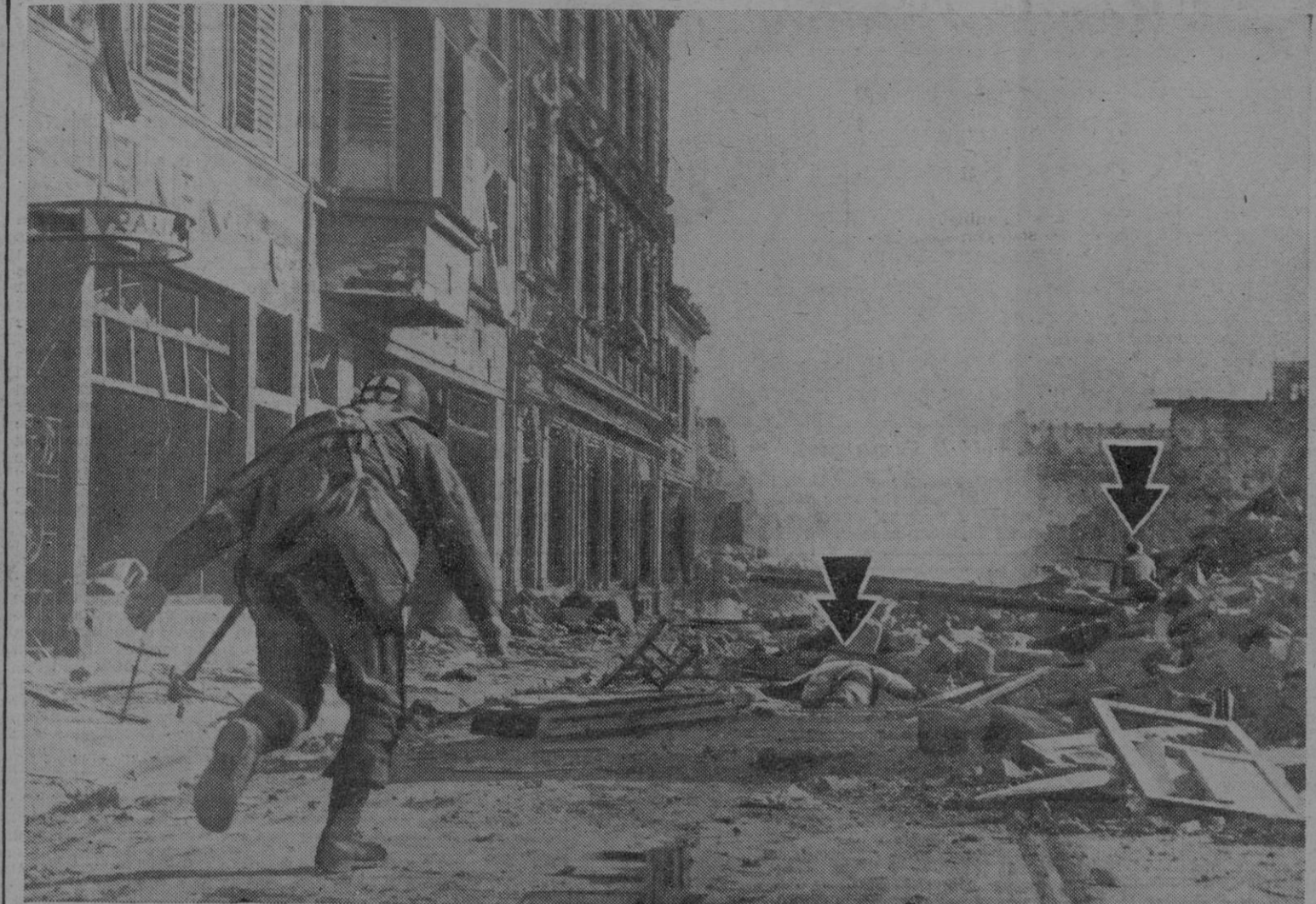
With smoke and dust still rising from the street in what's left of Saarlautern, Germany, a medic attached to the 26th Inf. Div. dashes forward to rescue an infantryman, wounded when a German shell exploded nearby. To the right, a bazookaman, dug-in in the rubble, sends a projectile into a German position to protect the advance of the medic who took advantage of the help to save the casualty.
