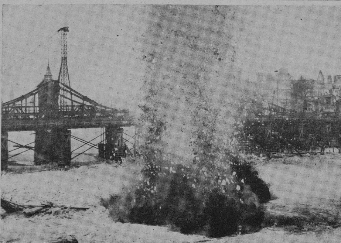
—Signal Corps Photo BREMEN BLAST: A charge of 80 pounds of TNT was set off recently in Bremen to relieve ice pressure against pilings of the Memorial bridge across the Weser river. The blast sent chunks of ice 200 feet into the air. This bridge is the only one left linking Bremen with the other side of the Weser.
