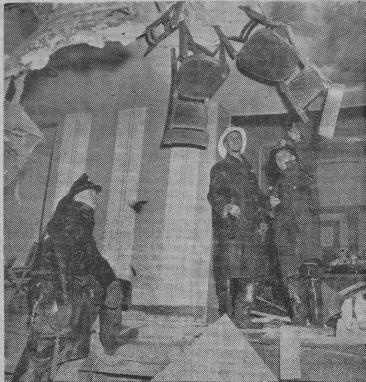
Firemen examine the wreckage after a terrific explosion wrecked a four-story factory building in Buffalo, N.Y. Three floors collapsed and a fourth is sagging. Two pedestrians near by suffered injuries.
