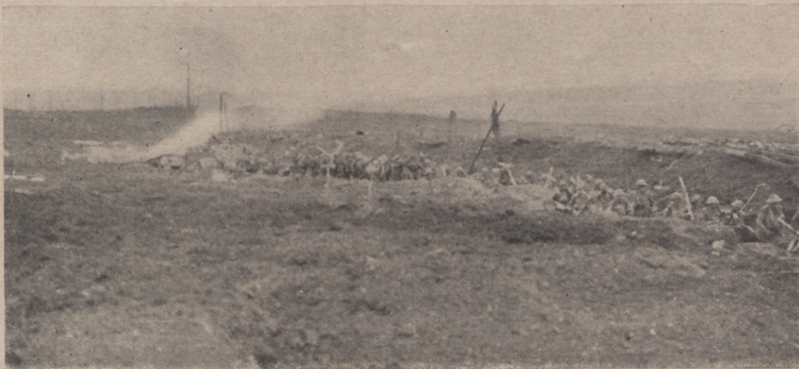
Looking towards Hooge. Supports coming up to the front.
