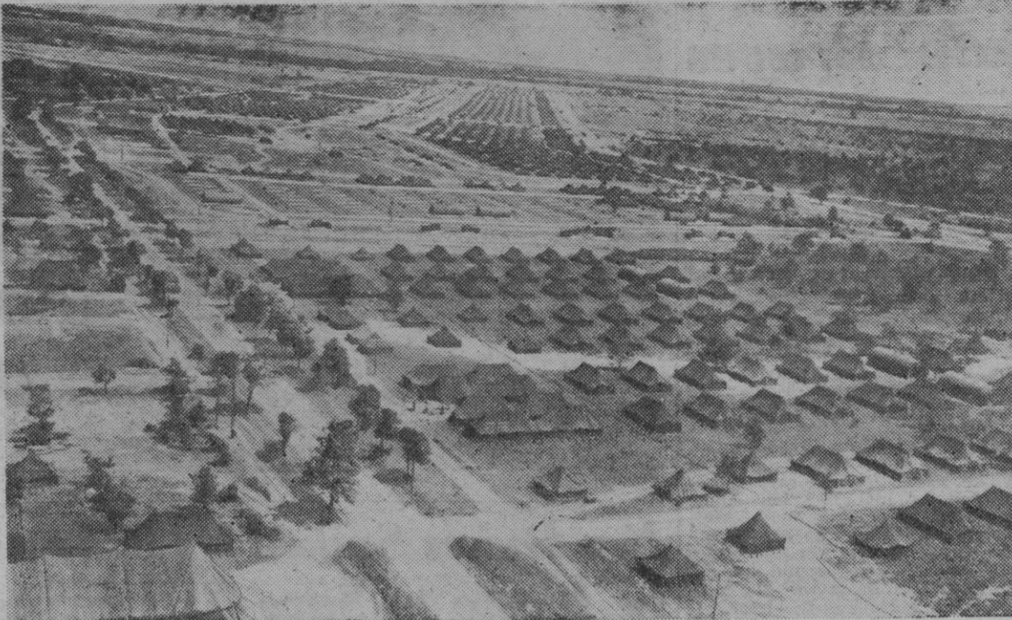
This is an aerial view of Camp Boston, ETO redeployment center in the Suippes sub-area of the Assembly Area Command. Thousands of U.S. troops are being processed at this and similar tent cities before shipment to the States.
