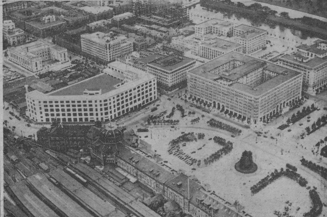
Here is the heart of Tokyo, capital city of the empire. The white building at the left is the Central Post Office, in the center foreground is the Tokyo Station and at the right stands the Marunouchi Building, hard-to-burn structures. Picture was taken in 1936.
