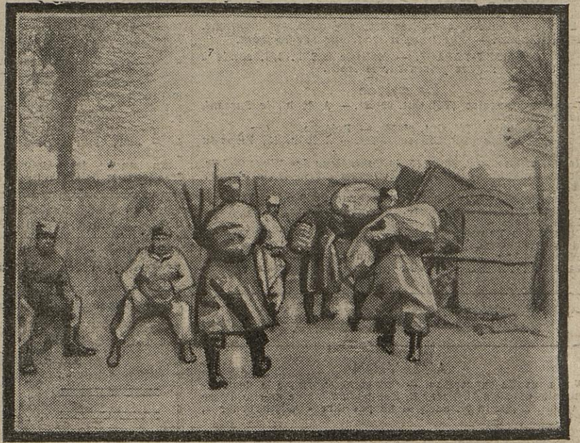
LA ROUTE FORTIFIEE
