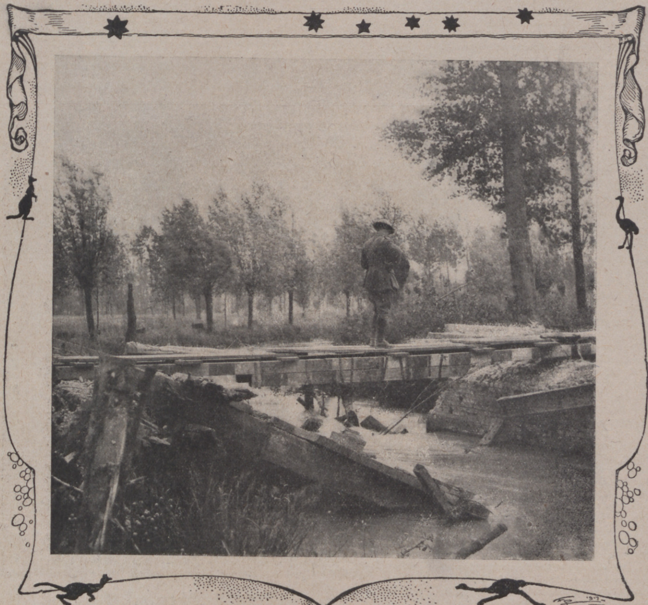
A temporary bridge to replace one destroyed by shell fire.
