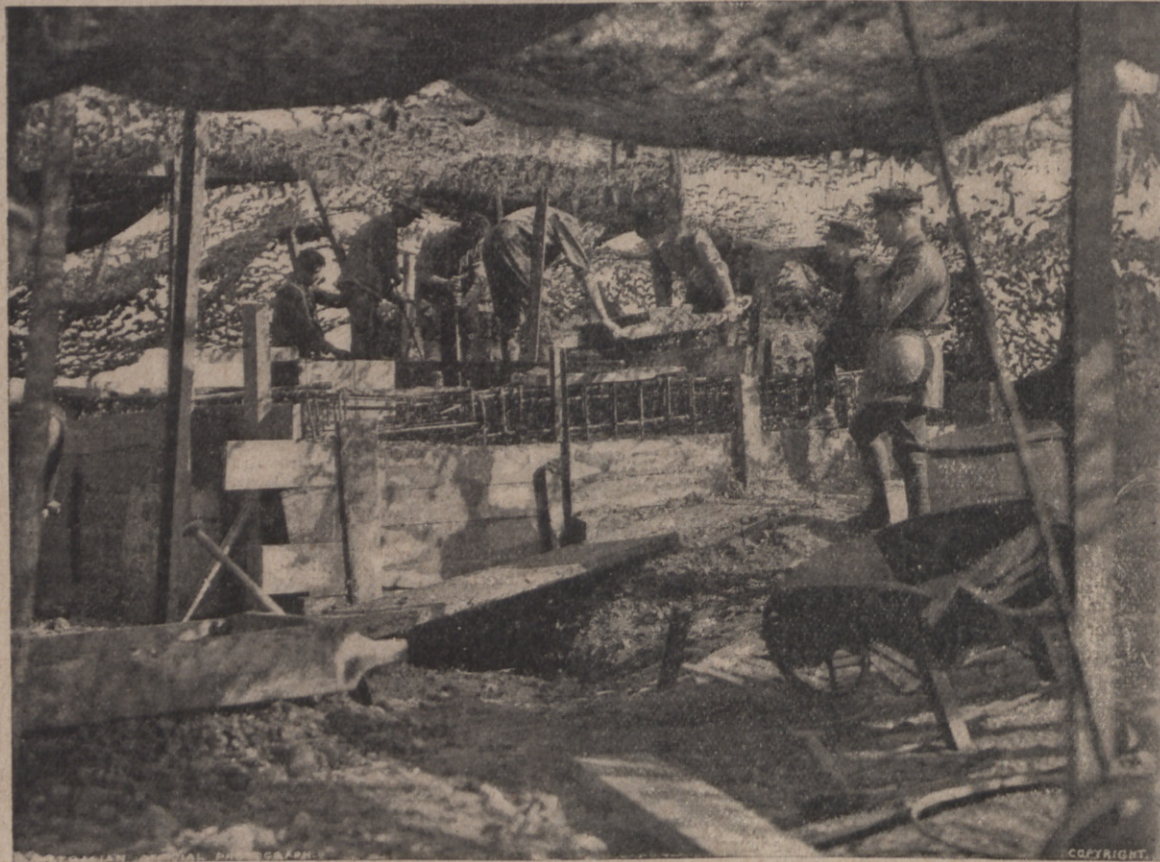
Building a reinforced concrete pillbox.
