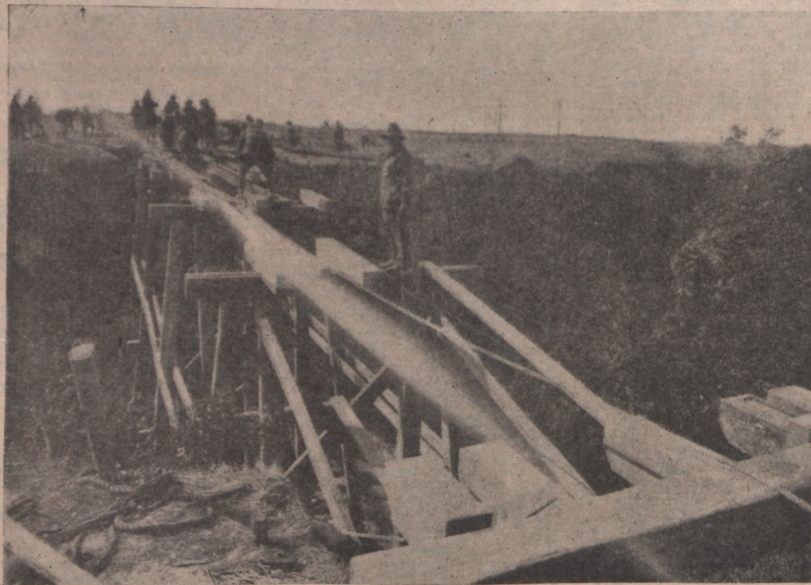
Timber trestle and a bridge built alongside destroyed arch bridge.
