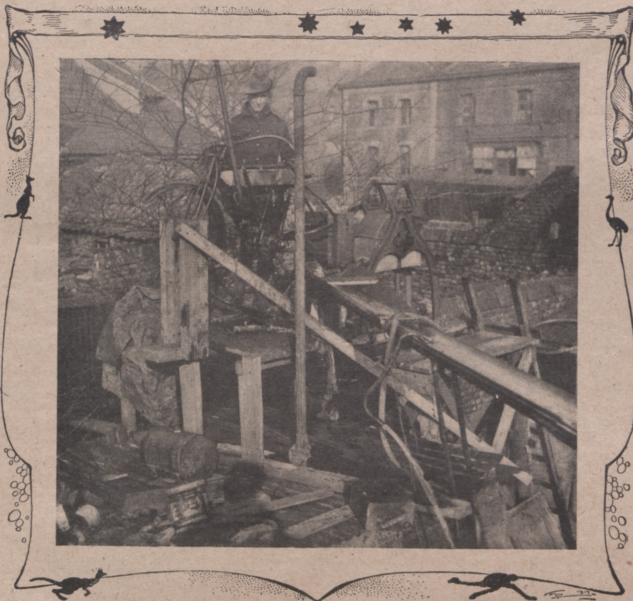
Ingenious Australian Miners. Salvaged motor cycle being used for power pumping plant.
