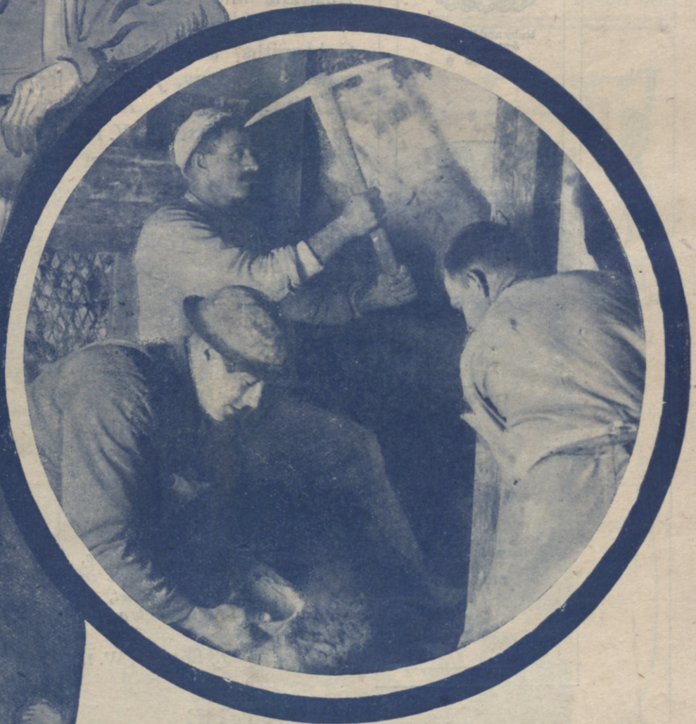
Australian Miners Constructing Dug-out.
