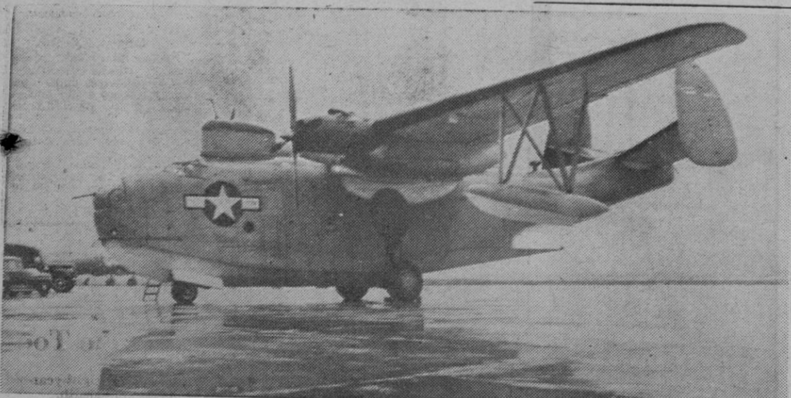
The largest amphibian plane ever built, the XPBM54, stands on the runway at the Glenn L. Martin plant at Middle River, Md. The giant 30-ton ship is a modification of the Martin PBM Mariner, twin-engined flying boat. The dual-purpose plane is able to take off from land or water.
