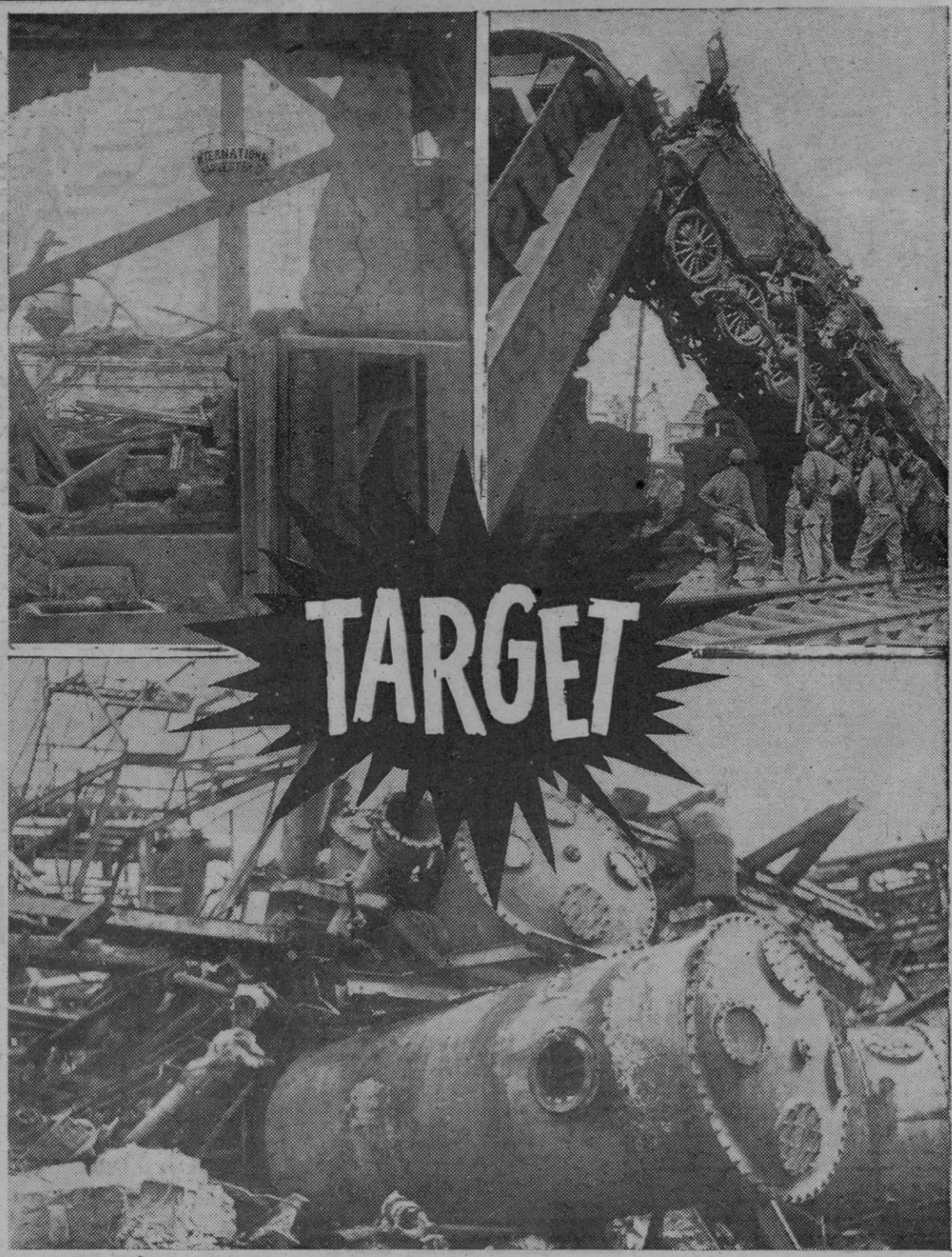
Strategical bombing of Reich had no favorites. International Harvester plant (upper left) and I. G. Farbenindustrie factory (below) at Ludwigshafen reduced to rubble. Arms train met fate at Munster.
