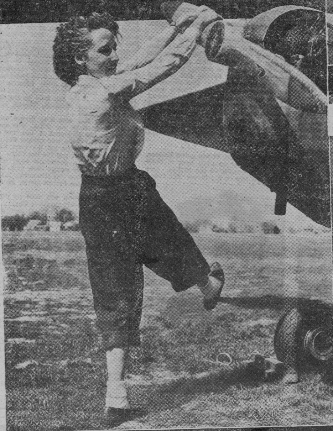
The large picture at the left shows Charlotte Ainsworth, president of the Smith College Flying Club, demonstrating the correct way to swing an engine over. (Above), Two Smith girls filling up the fuel tank of a trainer.
