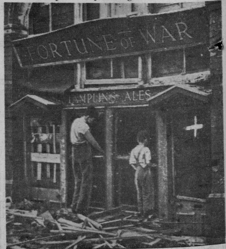
Two inquisitive youngsters stand on a pile of rubble to peer into the interior of the old public house, "The Fortune of War," which was damaged during the war by Nazi bombing attacks on Brighton, England.
