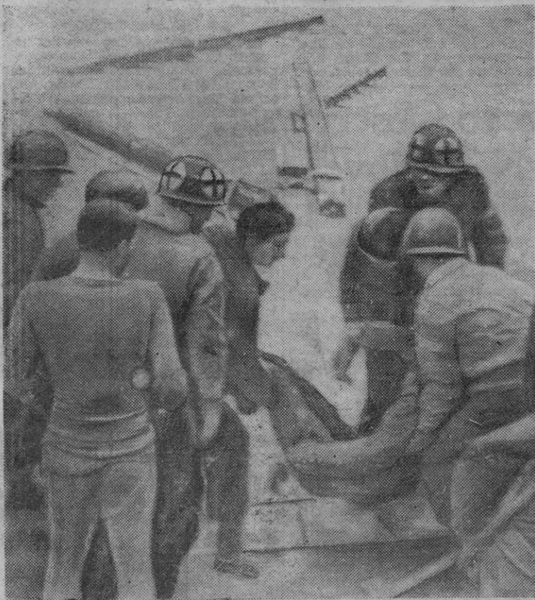
Helping hands take an injured engineer from the chill waters of the Rhine River near the collapsed Ludendorff Bridge at Remagen. His feet were crushed when the steel span caved in and he fell 75 feet to the swirling waters.
