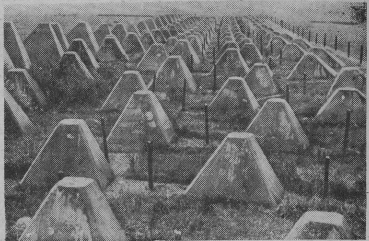
Concrete "dragon teeth" tank obstacles in the Siegfried Line near Lammersdorf, Germany.
