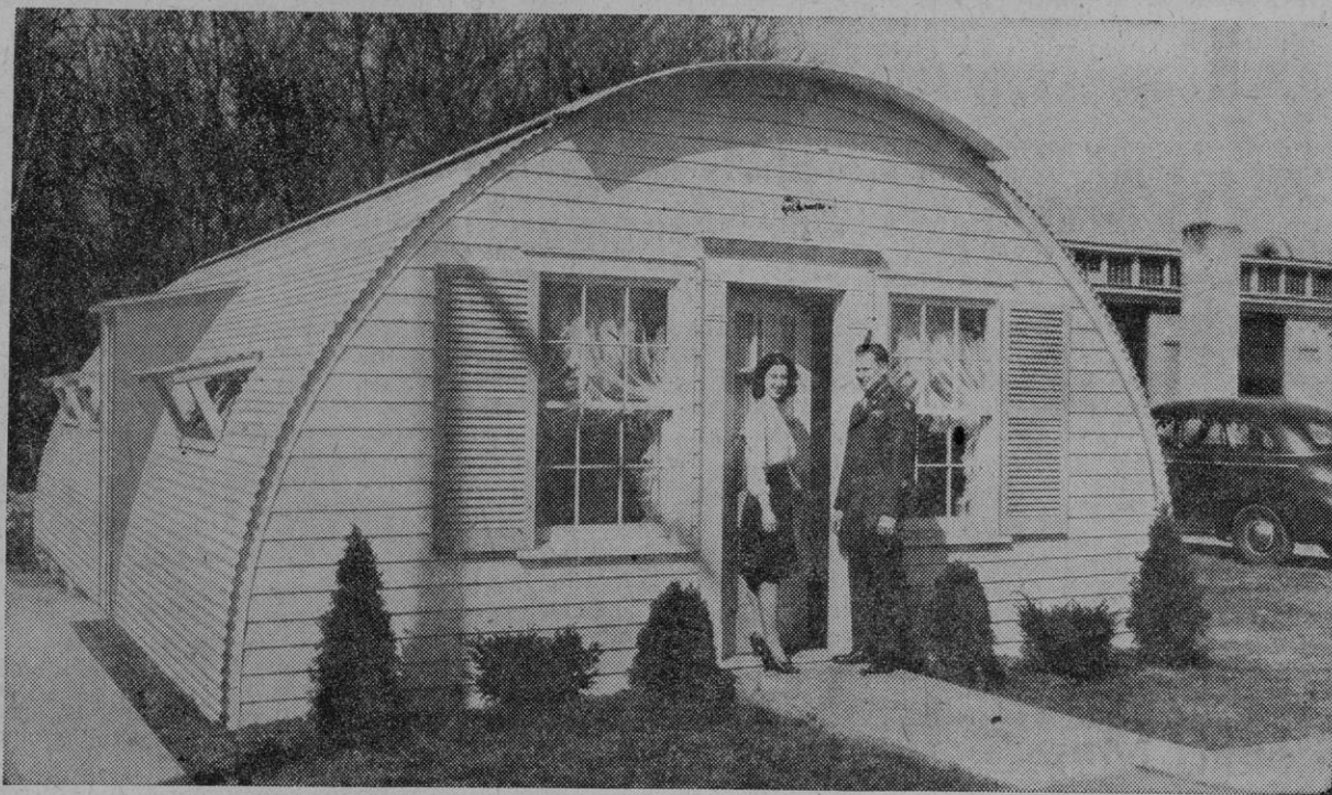
WARTIME quonset hut is being considered as an approach to solving the housing problem in Grand Rapids, Mich. Cost of hut, divided into living room, dining room, kitchen, two bedrooms and a bath, is $1,000.
