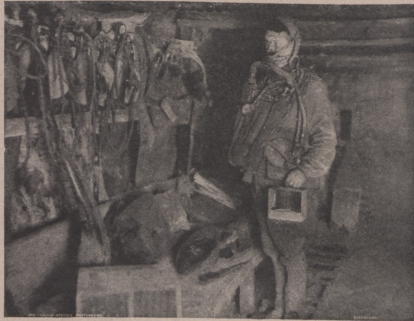
The Rescue Station in an Australian Tunnelling System. (Australian Official Photograph.)
