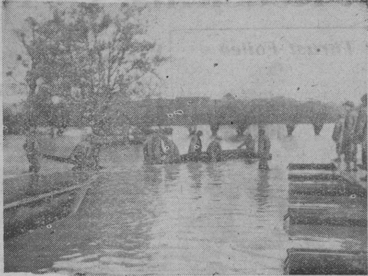
Combat engineers, up to their hips in the flood waters of the Moselle River (left), rush construction of a footbridge crossing an area inundated by the heaviest rain-
