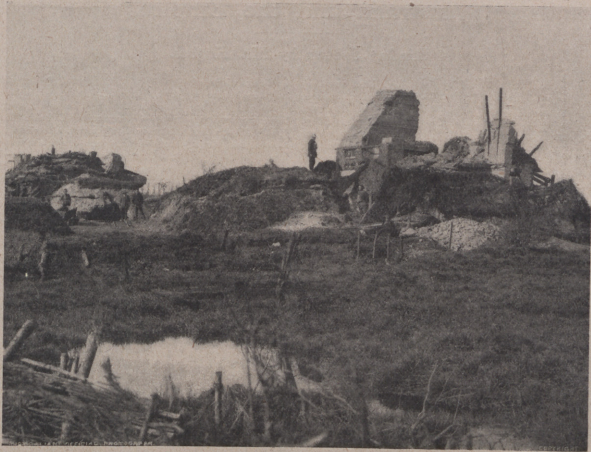
Summer Farm: Reinforced concrete shelters.
