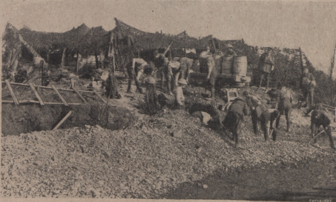
Building a reinforced concrete shelter.
