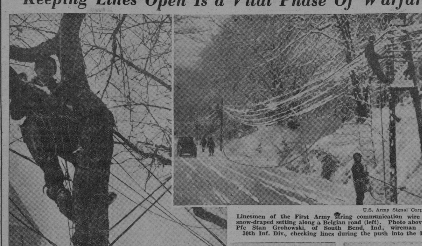
Linesmen of the First Army string communication wire in the snow-draped setting along a Belgian road (left). Photo above shows Pfc Stan Grabowski, of South Bend, Ind., wireman of the 30th Inf. Div., checking lines during the push into the Bulge.
