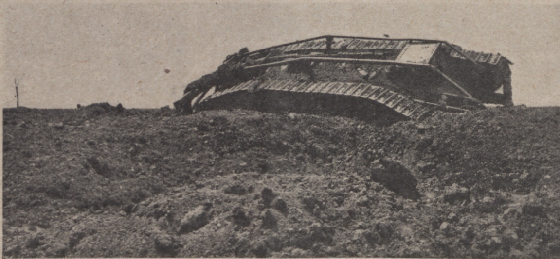
A derelict tank a few hours after it had been captured from the enemy. At the foot of the trees to the left is an occupied enemy machine-gun post.
