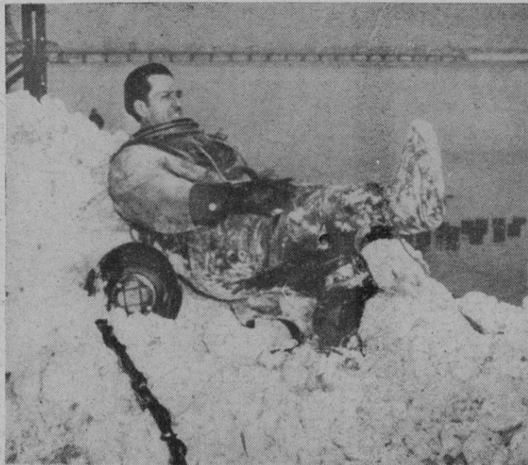
IRON SHOES: William Whyte, the Bronx, N.Y., dons a pair of underwater boots weighing 34 pounds which he will wear on the bottom of Port Newark, N.J., where he is helping to clear the way for ship launchings. Rubber mittens keep the diver's hands warm in winter so that he can feel his way around. —INS Photo
