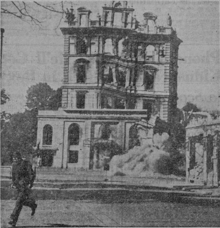
The work of clearing German cities of their ruins is under way. Here, a hotel in downtown Bremen begins to crumble from a blast of dynamite.
