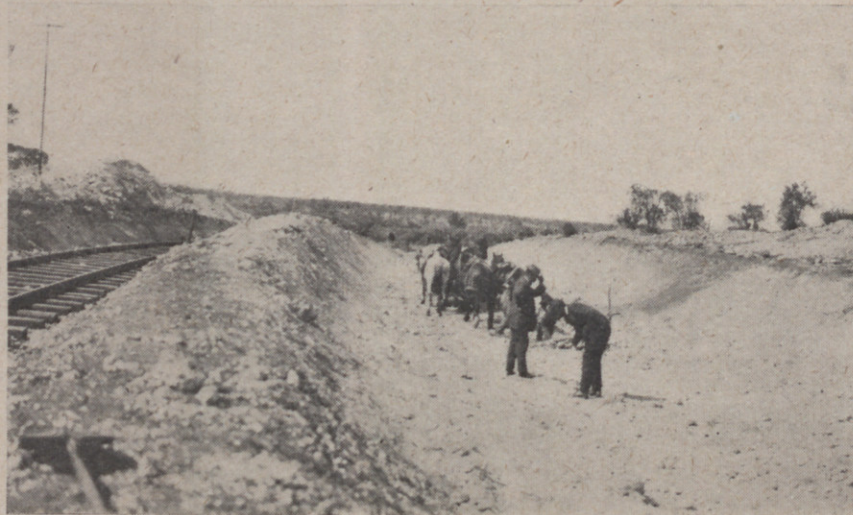
Cutting in progress with temporary deviation.
